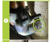
Scratch the pipe where it enters the home through the wall but before the elbow.
